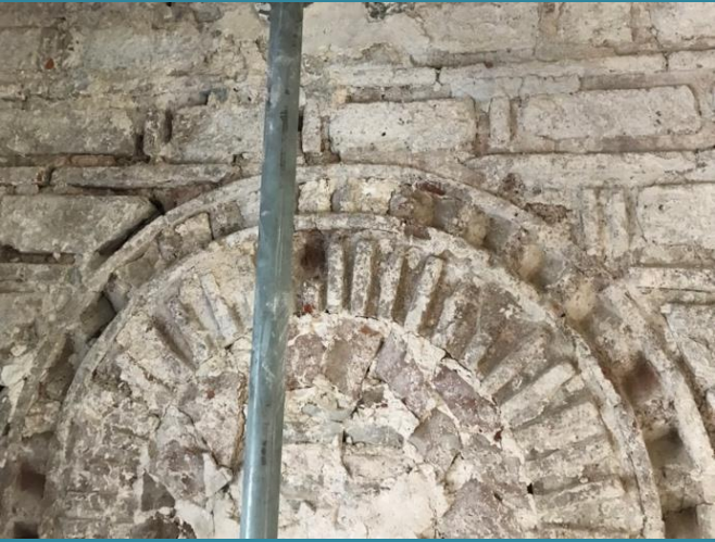
Byzantine masonry construction
