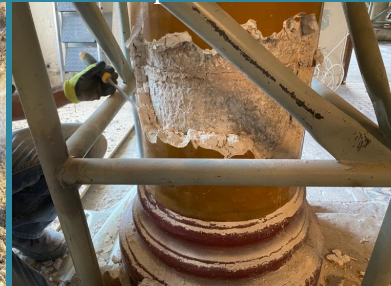
Stone pillar behind plaster
