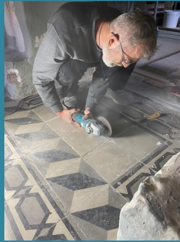
Removal of cement tiles
