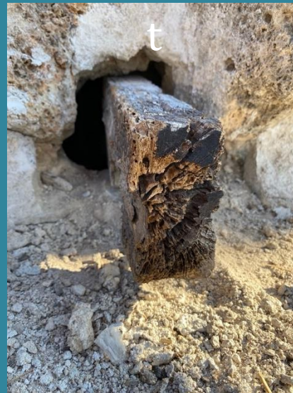
Wooden reinforcement
