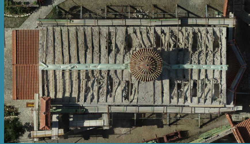
Documentation of roof system
