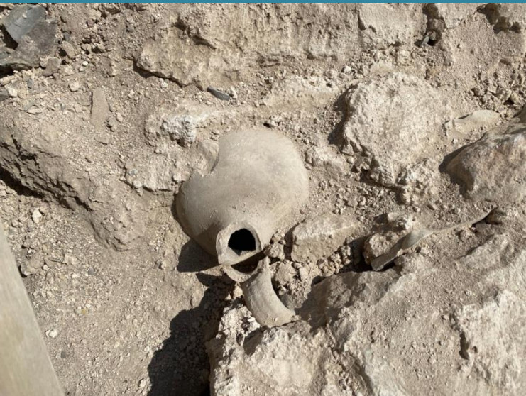
Ceramic jugs in the dome to enhance acoustics
