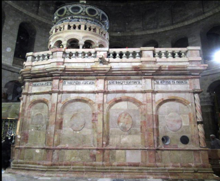
JUST AFTER THE REHABILITATION PROJECT
