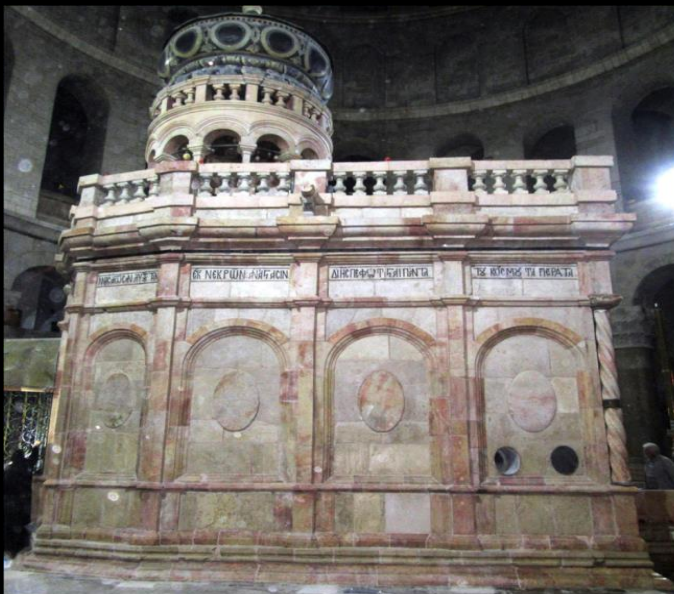
South façade, after the rehabilitation works
