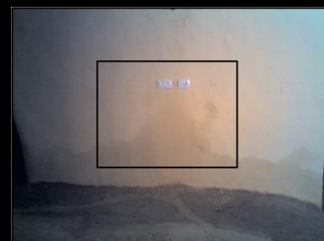
Detection of the actual rising damp front Remaining dampness
