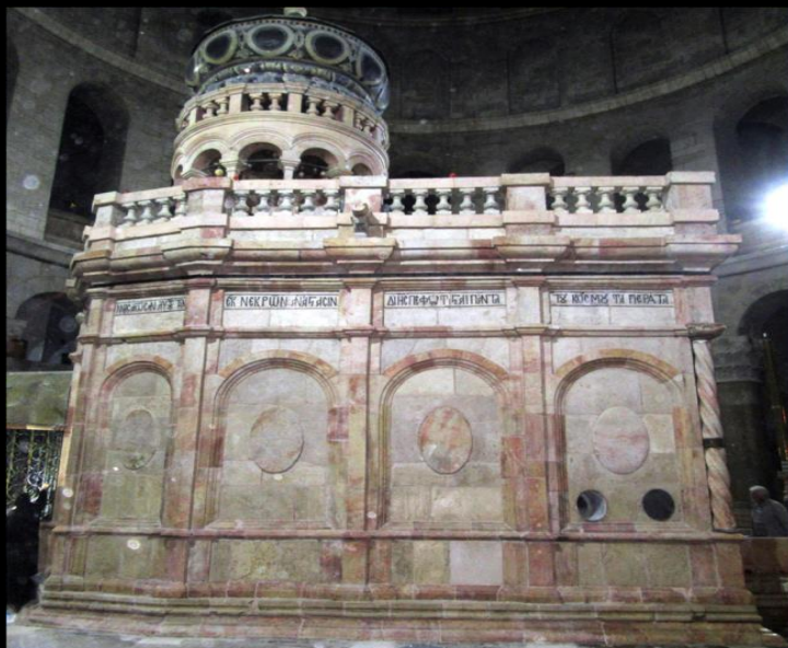
JUST AFTER THE REHABILITATION PROJECT
