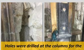
Holes were drilled at the columns for the installation of titanium anchors
