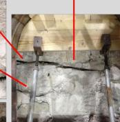
The finding of corroded iron support bars necessitates the use of titanium, as proposed by the NTUA interdisciplinary team, in order to avoid such phenomena and ensure the longevity of the structure
