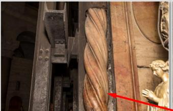
Cause of the deformation: Deterioration of the mortars & masonry swelling:
