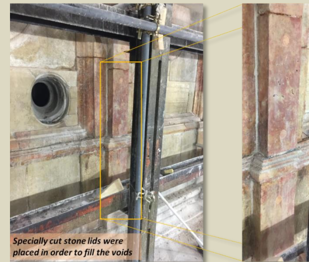
Holes were drilled at the columns for the installation of titanium anchors
