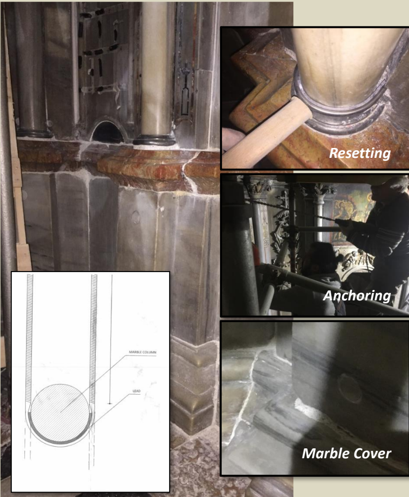
Plan for anchoring of columns in the interior of the Chapel of the Angel (by Assist.Prof. Ch.Mouzakis)
