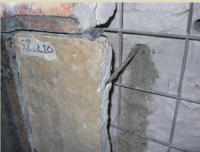
Process of stone slabs reassembly
