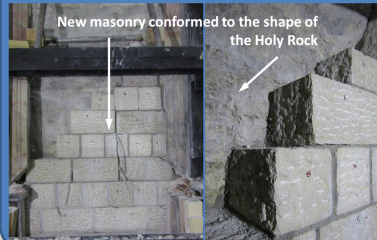
Interior historical masonry after removal of slabs
