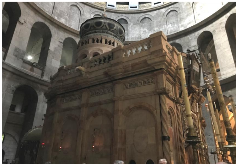
Figure 1. The Holy Aedicule of the Holy Sepulchre as it stands today, viewed from the south.
